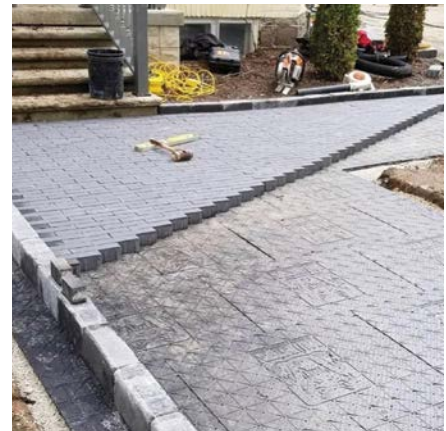
"No more 9 to 10 inches of excavation! When you're excavating material and have to go dump it. Absolutely there's savings there."
