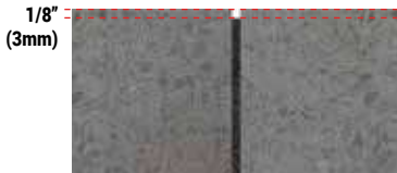
PAVERS OR NATURAL STONES WITHOUT CHAMFER
